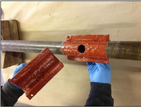
Fig. 7. Center the coupling directly over the hole. The edge of the hole must be at least two inches from the ends of the coupling.
