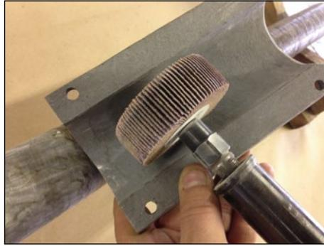
Fig. 5. Abrade the inside radius and the flanges of the coupling.
