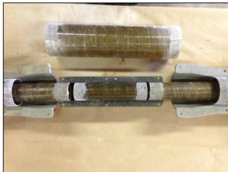
Fig. 14. When repairing contained lines, use containment pipe one size larger than usual. Align the wing-nuts parallel to the pipe axis to permit the containment to slip over the repair coupling.
