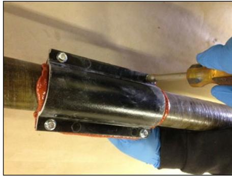
Fig. 8. Join the coupling halves. Tighten bolts evenly. A bead of adhesive should be visible between the pipe and the ends of the coupling and between the flanges.
