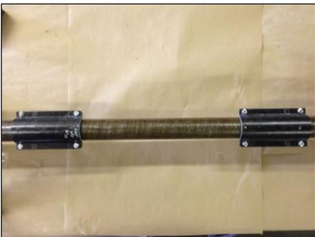
Fig. 13. For damaged areas over 10 inches in length, join the replacement nipple to the existing line with either full-size couplings or half-couplings.
