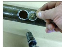
Fig. 2. Delaminated areas must be removed from the pipe. Small delaminations can be removed with a hole saw.
