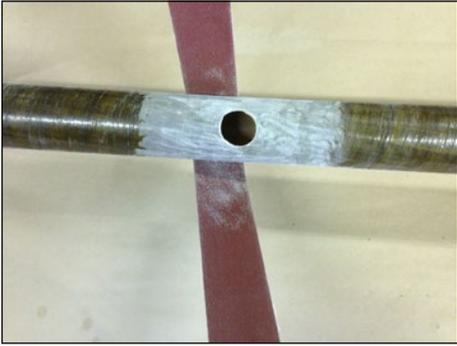
Fig. 4. Abrade all bonding surfaces on the pipe with emery cloth or a flapper sander.
