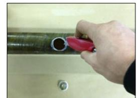
Fig. 3. Clean cut edges thoroughly and remove any loose material.
